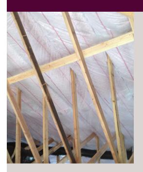
Owens Corning's unvented attic uses a proprietary netted and blown-in fiberglass insulation system that offers a number of benefits compared to other approaches.
